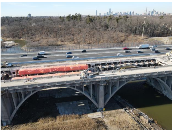
FEBRUARY: Phase 1: Demolition and removal of the existing QEW bridge deck.
