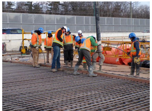
MARCH: Existing QEW bridge, first concrete pour for the new deck.
