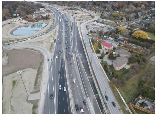
NOVEMBER: Opened up the QEW westbound on-ramp from Mississauga Road.
