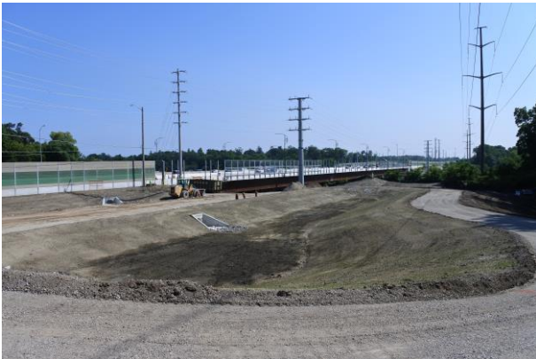
JUNE: The stormwater management pond at Stavebank Road-Premium Way completed.
