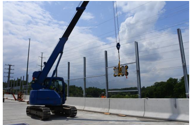
JUNE: Installation of the bridge clear noise wall panels.
