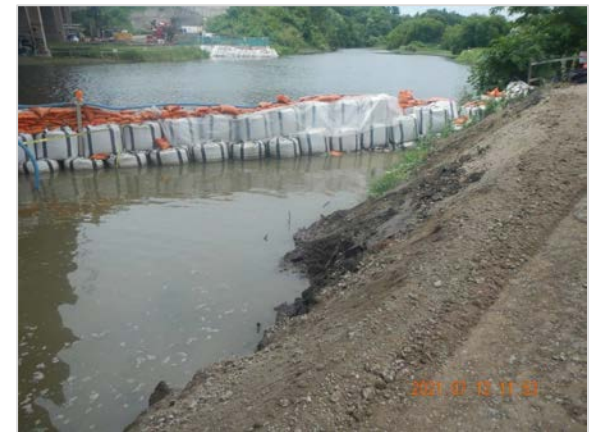
Isolating the work area for the new Credit River Bridge
