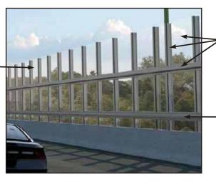
Embedded wire mesh (or, filaments) provide fragment retention, preventing fragments from falling to the river below in the event of a collision.
